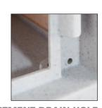
**COMPARTMENT DRAIN HOLE** SITS NEATLY OUT OF SIGHT **BEHIND THE DOOR\***
